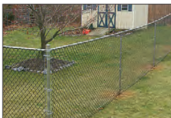
Chain Link Fence
