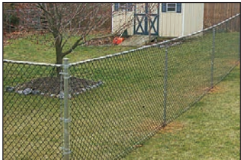
Chain Link Fence
